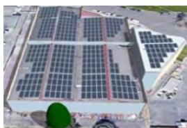
KCHI (Rubî) 185 kWp
